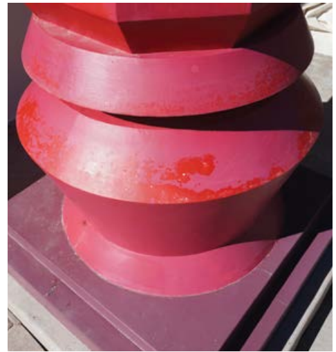
Restoring the dramatic gateways with a high-performance protective coating was overdue, as the paint on the intricately ornamented arches and support columns was significantly faded, chipping and flaking.
