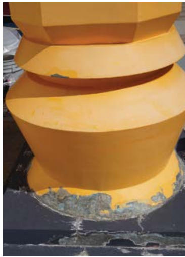
Restoring the dramatic gateways with a high-performance protective coating was overdue, as the paint on the intricately ornamented arches and support columns was significantly faded, chipping and flaking.
